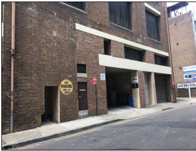
Figure 23: The utilitarian rear elevation of the site.
