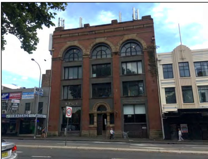
Figure 16: The primary southern elevation of the subject site.
