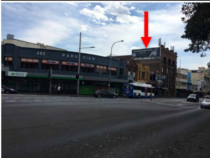
Figure 38: Looking east along Broadway towards the subject building.
