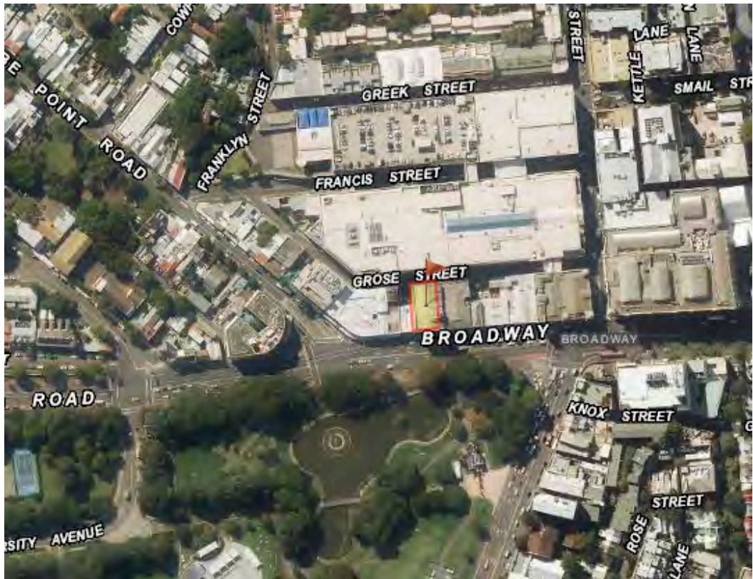
Figure 32: Aerial photograph over the site and the surrounding area.
