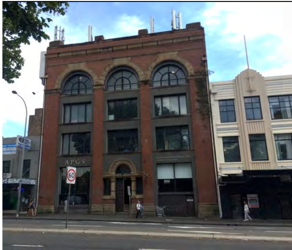
Figure 2: The primary southern elevation of the subject site.
