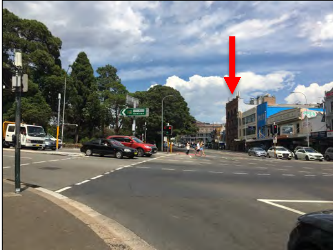
Figure 37: Looking west along Broadway towards the subject building.
