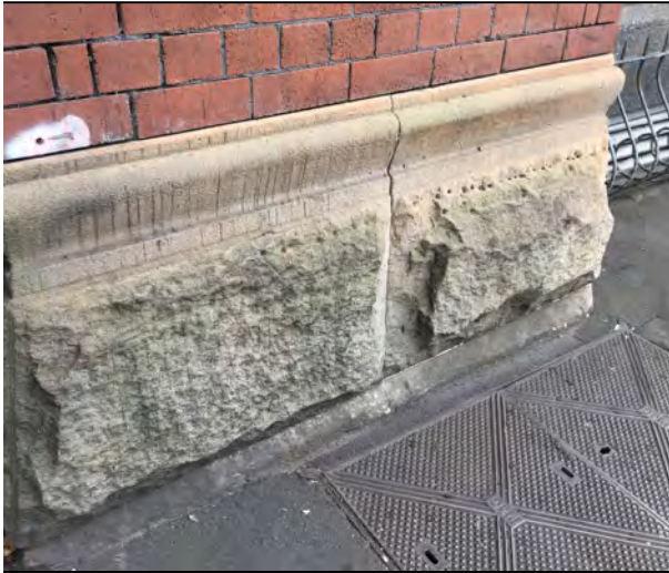
Figure 4: The sandstone base on Broadway.
