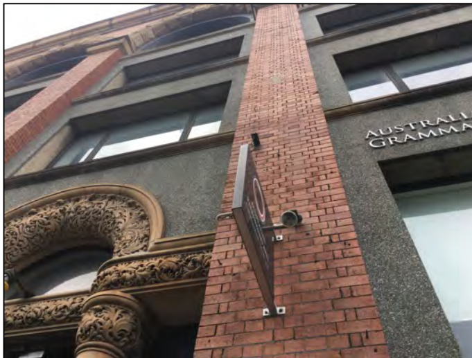
Figure 21: Looking up the face brick column on the primary elevation.
