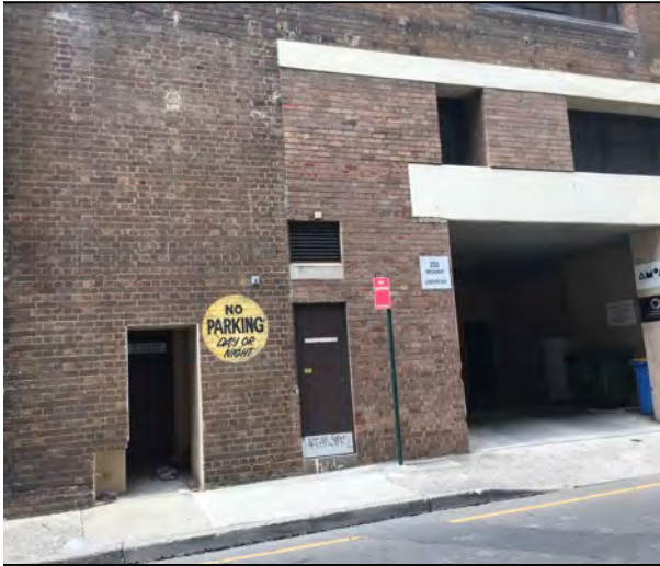
Figure 10: The utilitarian rear elevation of the site.
