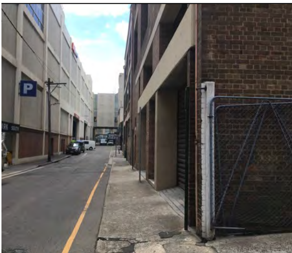
Figure 11: The western elevation of the rear entry on Grose Street.
