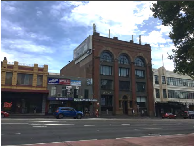
Figure 17: The southern elevation showing part of the western elevation.
