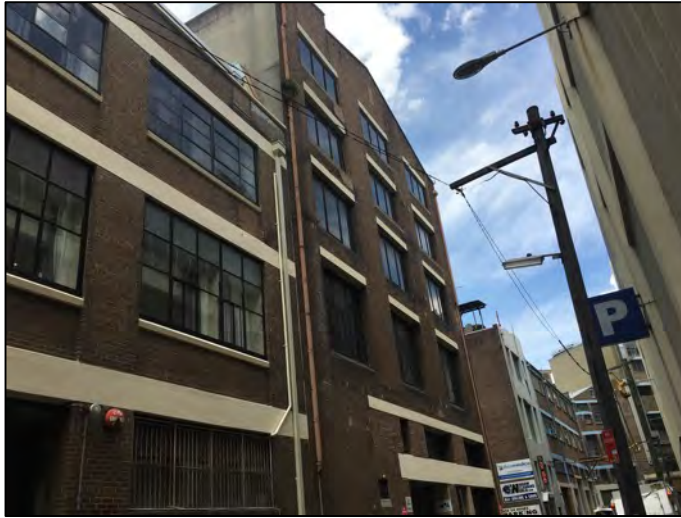
Figure 22: The utilitarian rear elevation of the site.
