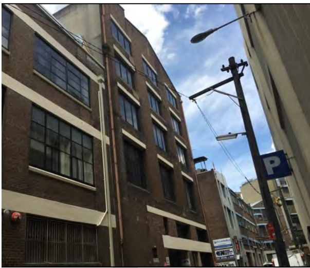
Figure 8: The utilitarian rear elevation of the site.
