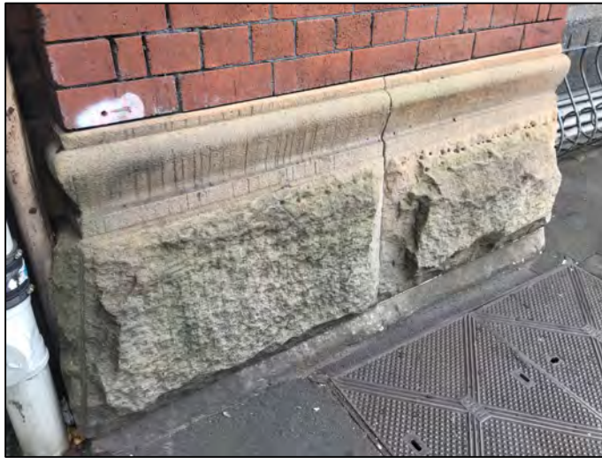
Figure 18: The sandstone base on Broadway.
