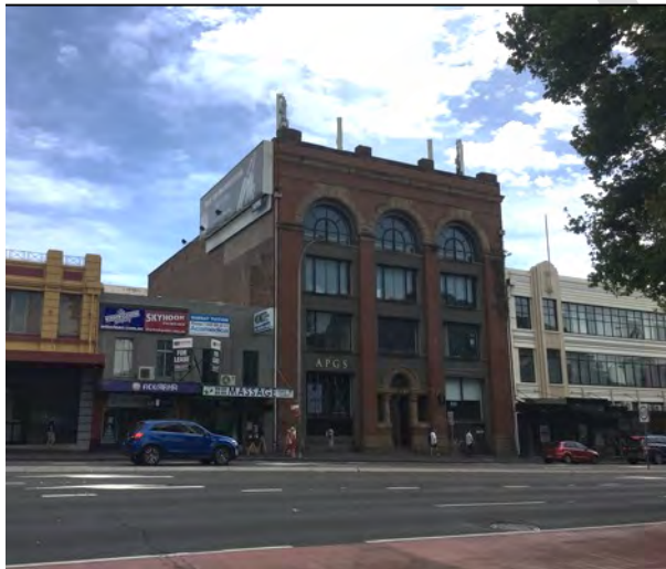
Figure 3: The southern elevation showing part of the western elevation.
