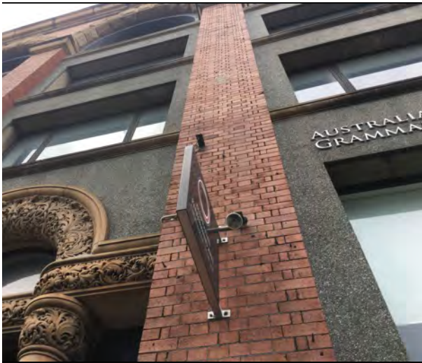
Figure 7: Looking up the face brick column on the primary elevation.
