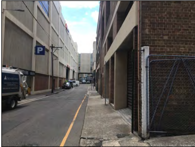
Figure 25: The western elevation of the rear entry on Grose Street.
