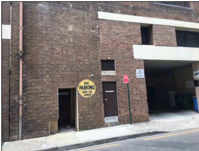
Figure 24: The utilitarian rear elevation of the site.
