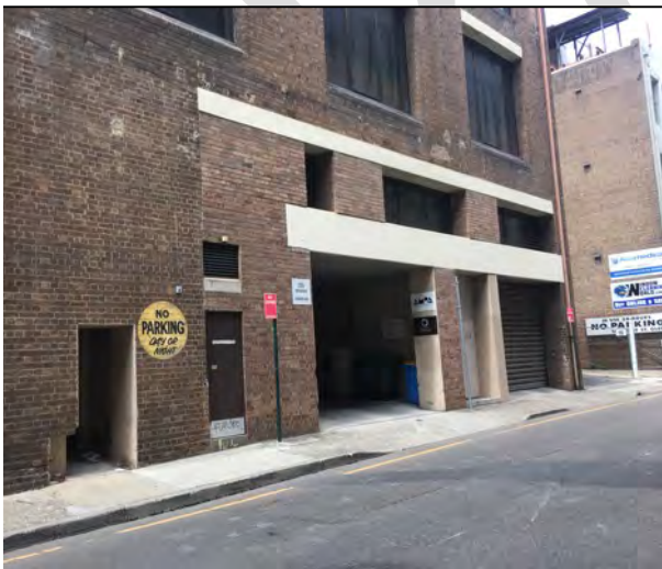
Figure 9: The utilitarian rear elevation of the site.
